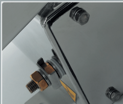
Earth stud with cable anti-rotation bracket
