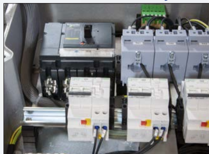
Built-in /magneto thermal circuit breakers
