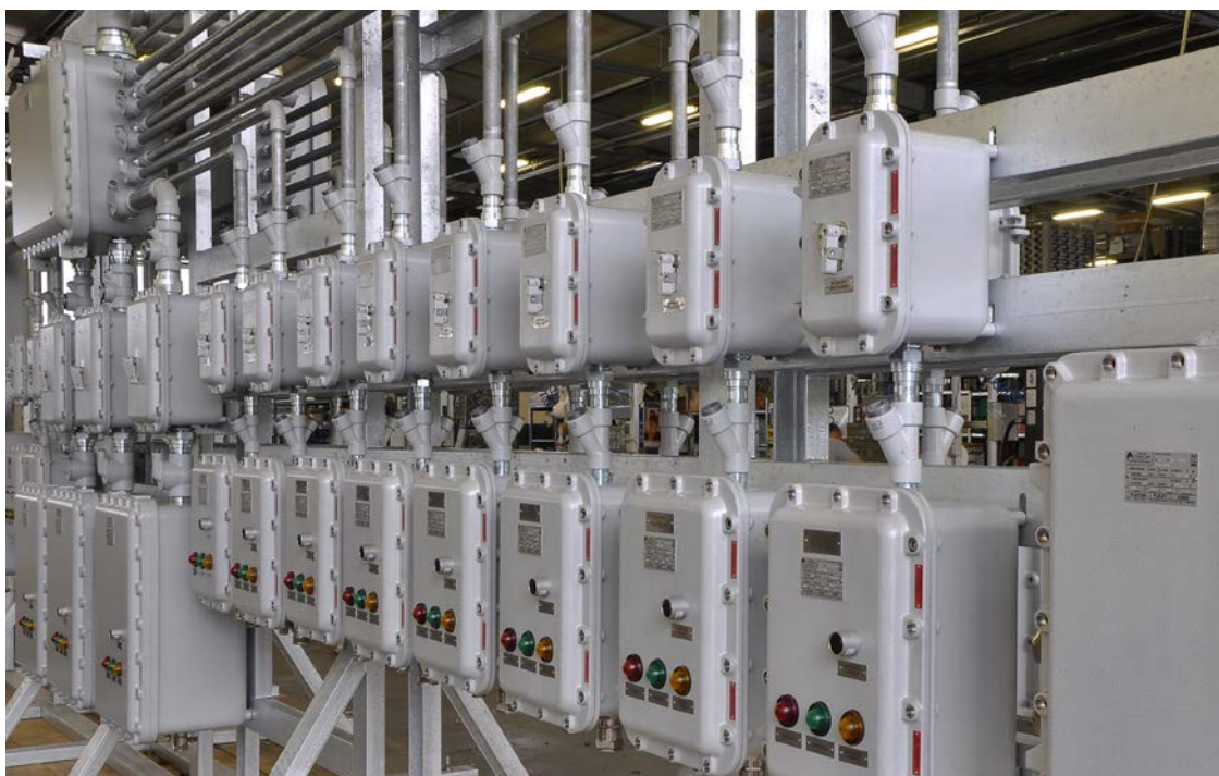
Fig. 16 Control panel with double-fronted installation made on the customer's specifications
