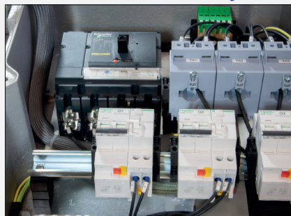
Built-in /magnetothermal circuit breakers
